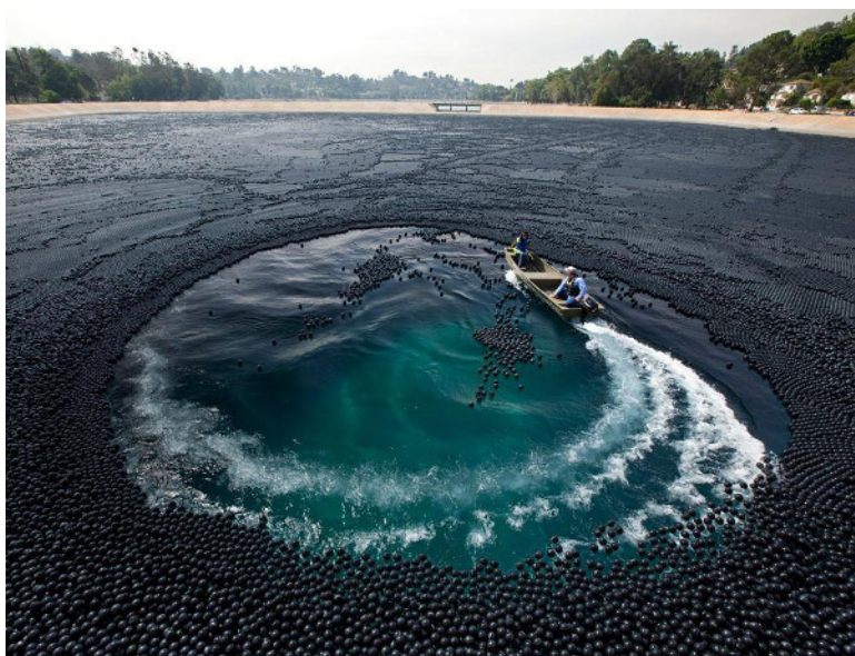
Figure 3.11: Dark polyethylene (PE) spheres at the air-water interface to reduce the level of bromate in Ivanhoe clean water reservoir. Image taken from [Ivanhoe, 2011].
